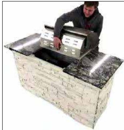
Placing the Grill Head
