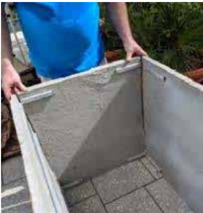
Assembling the Frame
